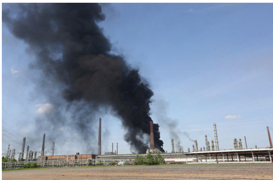
Shell Refinery Wesseling
