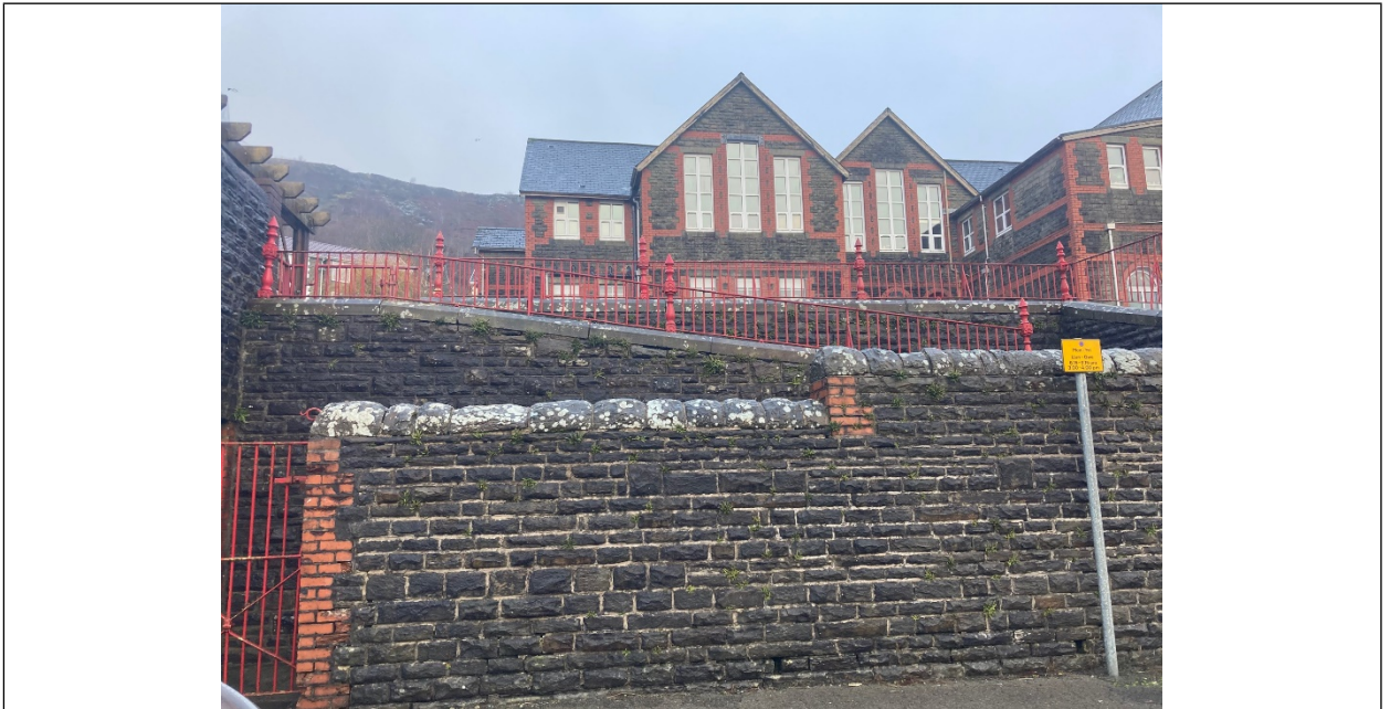
The view of the existing school building from Darran Terrace.
